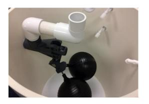
SUFFICIENTLY WRAP STEM OF NEW KERICK VALVE ASSEMBLY WITH TEFLON® TAPE, THEN SCREW SNUGLY INTO TANK SIDEWALL. ROTATE TOP PIPING AS SHOWN.
