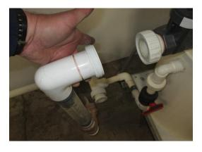
REMOVE FLOW METER AND SOLENOID VALVE ASSEMBLY.
