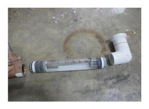
CAREFULLY REMOVE FLOW METER FROM OLD PIPING.
