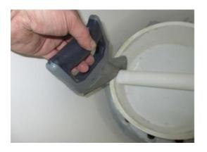
CUT OLD INTERNAL SPARGER PIPING AND REMOVE.
