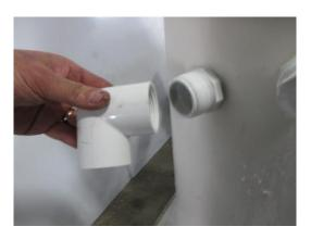
INSTALL THREADED BUSHING AND T X T 90° ELBOW.
