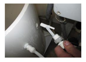
REMOVE/UNWIRE LEVEL SWITCH AND SOLENOID.
