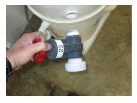
REMOVE GATE VALVE FROM CHLORINATOR.
