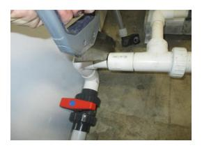
CUT TO REMOVE ADDITIONAL SUPPLY PLUMBING. LEAVE SEVERAL INCHES FOR ATTACHING INLET PIPING.
