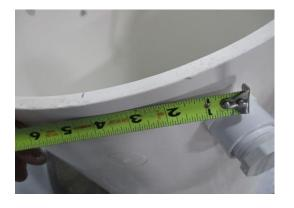
MEASURE OVER 4", DOWN 5-3/4", AND MARK LOCATION FOR NEW FLOAT VALVE.
