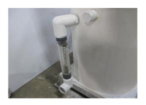
INSTALL T X S 90° ELBOW ON BOTTOM OF FLOW METER & THREAD ALL PIECES TOGETHER; POSITION FLOWMETER AS SHOWN.
