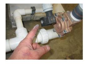
REMOVE NUT FROM SOLENOID COIL.
