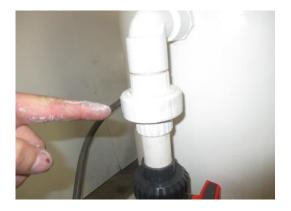
LOOSEN UNION AND REMOVE PIPING.
