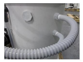
Using 7/8" hole saw, drill two 7/8" holes into enclosure for conduits. Install fittings into holes. Pull the level switch wires into the enclosure and secure conduits in the fittings. Chlorinator images: Accu-Tab<sup>®</sup> 3070 shown on left; Accu-Tab<sup>®</sup> 1030 shown on right.
