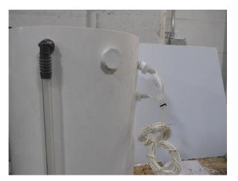
4. Install bushing in conduits if not already installed. Pull the wire of one switch through each conduit and twist conduits onto switches, being careful not to break or change the position of the switches.
